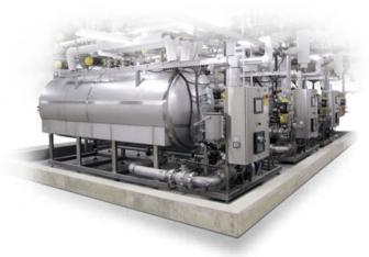
Three 1,750 gallon per cycle effluent decontamination system installed at the Ohio Agriculture Research and Development Center, The Ohio State University.
