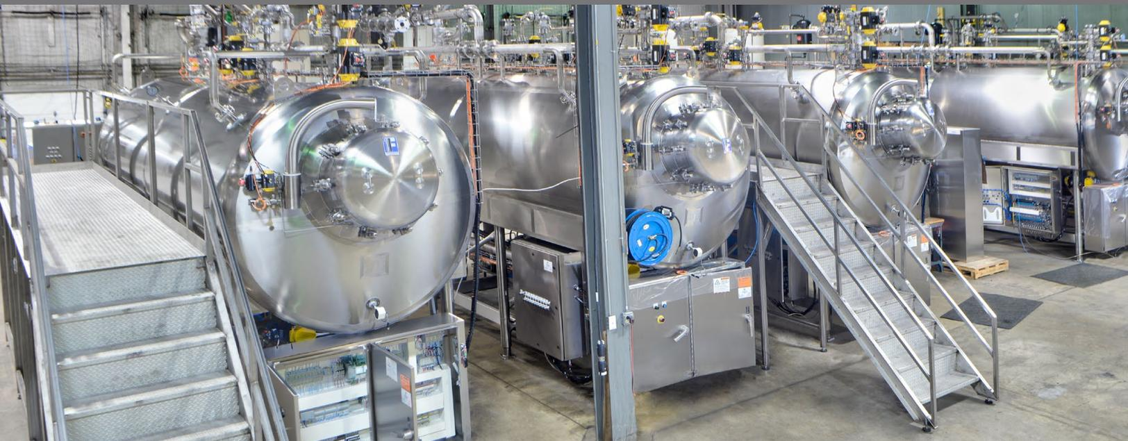
BSL-4 62,000gpd Effluent Decontamination System—USDA Plum Island, 2017.
