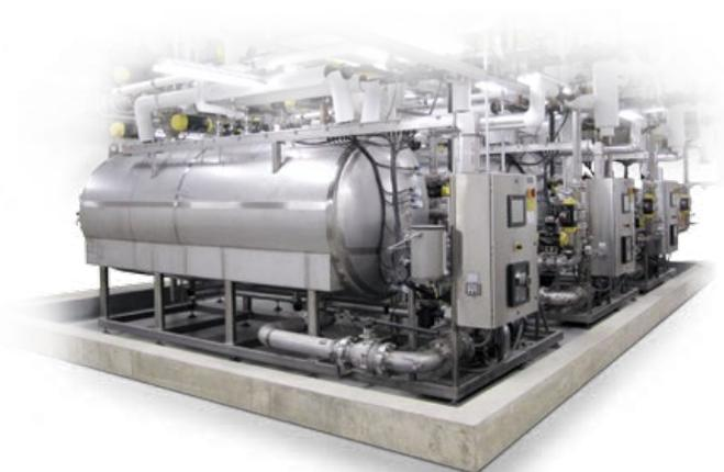
*Three 1,750 gallon per cycle effluent decontamination system installed at the Ohio Agriculture Research and Development Center, The Ohio State University.*
